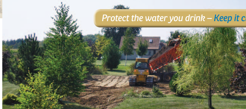
Yards may need to be re-worked to divert runoff from sinkholes, fractures or old wells. Here a man-made pond collected polluted runoff from the surrounding fields, yard and road ditch, but never held water for long. It drained through a bedrock fracture, repeatedly contaminating groundwater. The pond had to be filled-in and the yard graded to stop the contamination.
