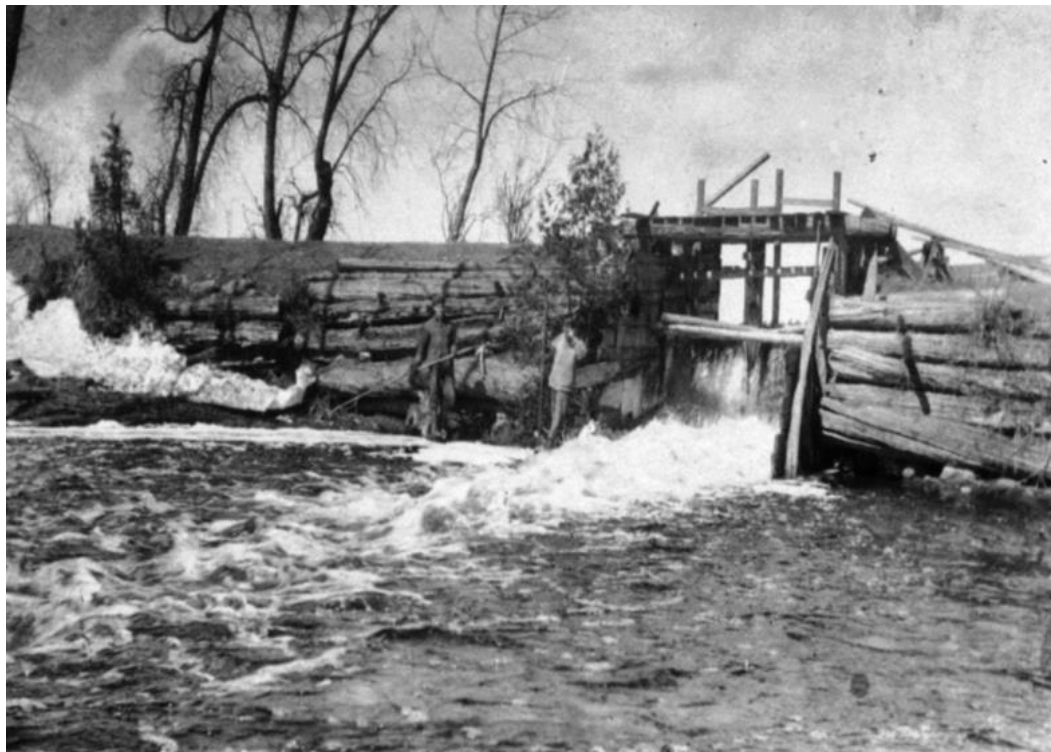
Figure 1-2. Forestville Dam in 1918
