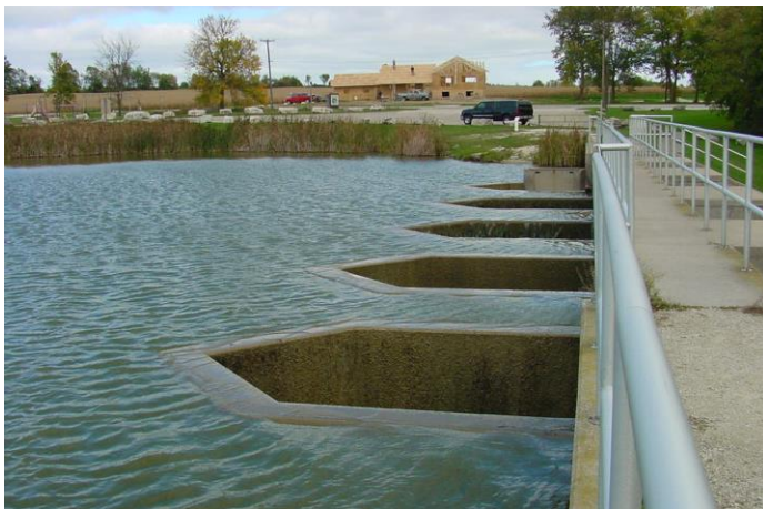
Figure 1-5. Dam Overflow Spillways
